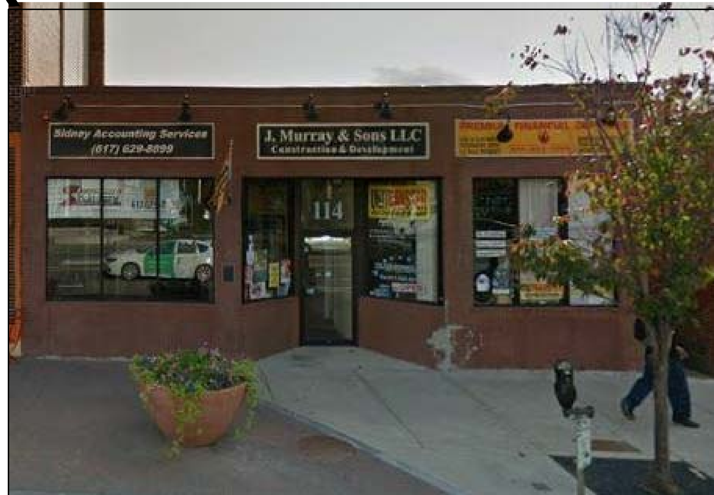
EXISTING BUILDING LOCATED AT 114/ 116 BROADWAY
